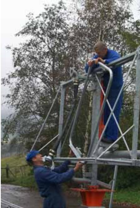
17. Turn the locking bracket on the central pendulum bearing to the centre support. This prevents the assembly from oscillating and the boom arms are easier to mount.
