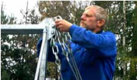
18. Fix the chain links of the cables to the pendulum center part. Adjust length variations of the cables with these links.
