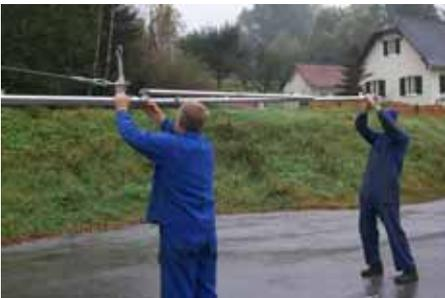
27. The last of the boom pipes cannot be folded in. They are pushed into the coupling, hooked up to the wind bracing, and coupled. Cable no. 6 is connected to the last pipe.
