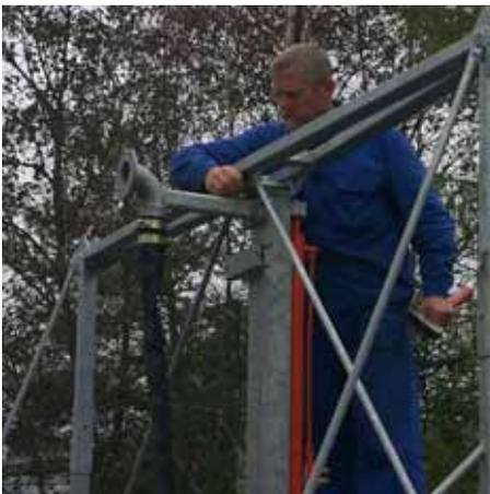
16. Mount the pendulum center part with the horizontal wind bracing facing backwards on the center support with the pin. The guide frame is re-mounted on the center support.
