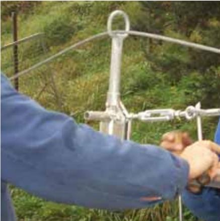
26. With the turnbuckles on the cables, the boom pipes can be adjusted in a level position.
