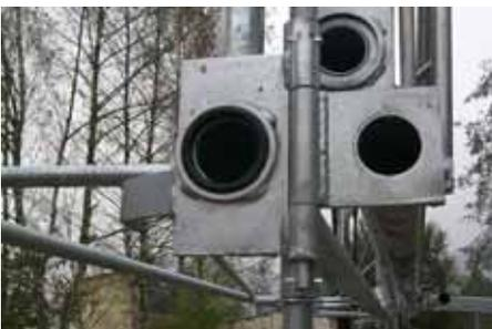
21. Rubber sealing rings are fitted into the pipe flanges.
